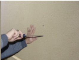
STEP 2. Start fasteners in wall.
