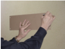
STEP 1. Mark wall with supplied template.
