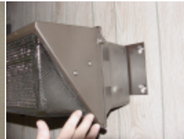
STEP 3. Hang wall pack using keyhole slots.
