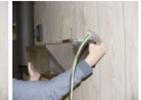
STEP 5. Connect wall pack to external j-box.
