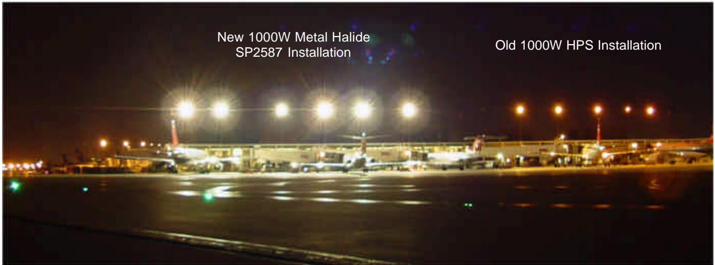
More than twice the light with Esco Lighting's computer designed forward throw SP2587 reflector system.
